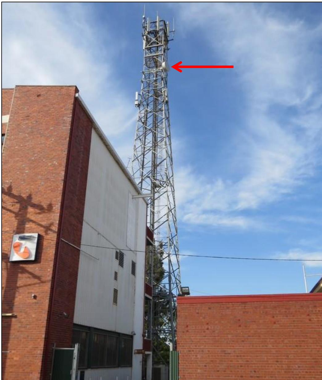
Figure 1: View looking to site from Richardson Street. The dish proposed to be replaced is shown. The existing 1.2m dish will be replaced by one with a diameter of 1.8m – the difference is not expected to be obviously noticeable from ground level, given the height of the tower (photograph from RFNSA database, www.rfnsa.com.au )
