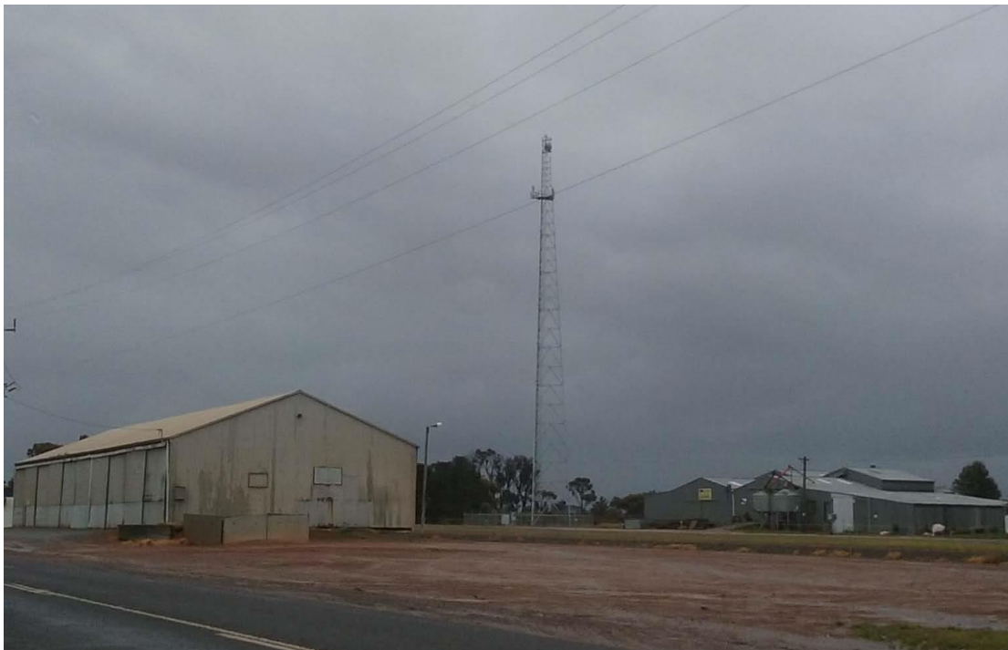
Example of 60m lattice tower (In Tambellup).
