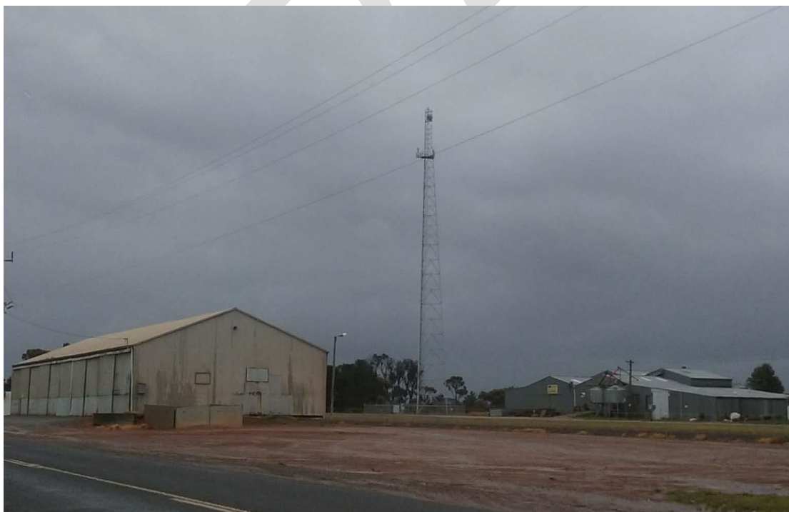
Example of 60m lattice tower (In Tambellup).
