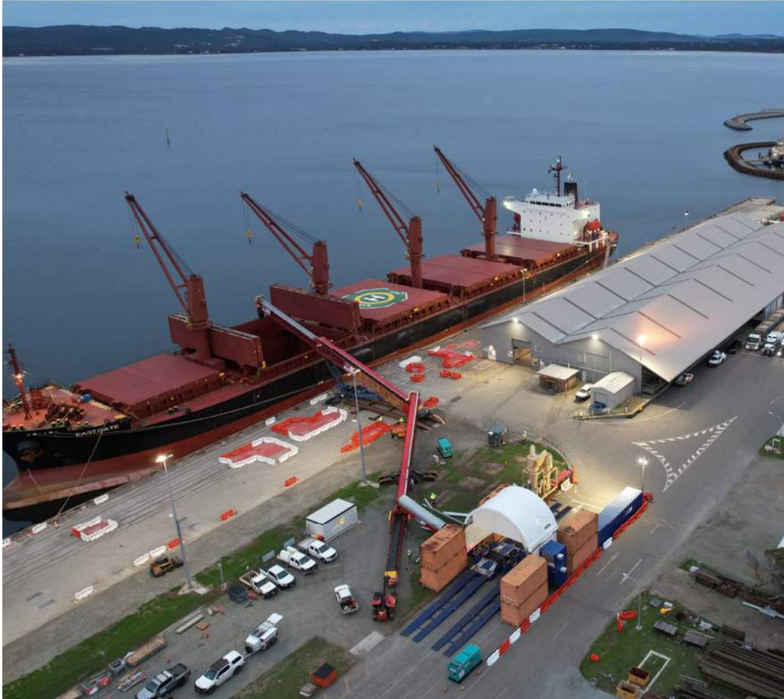
Figure 8 Port of Albany Grain Handling
