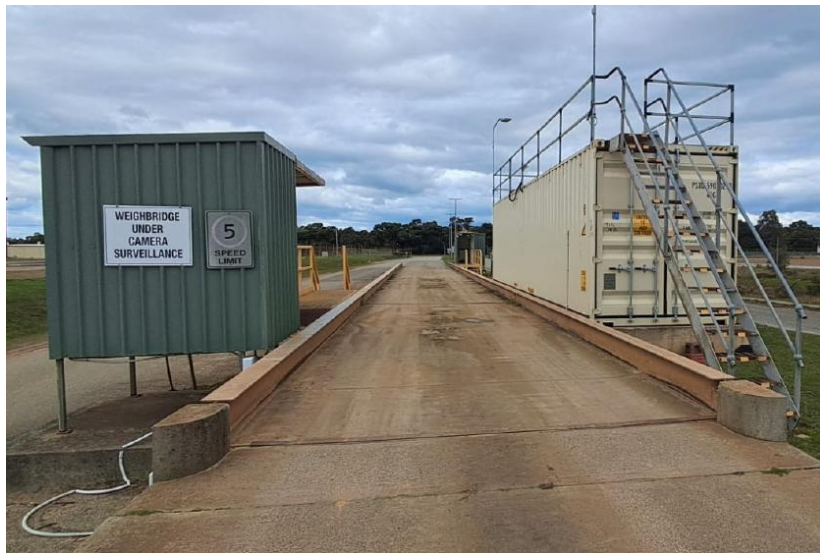
Figure example of weighbridge and sampling hut
