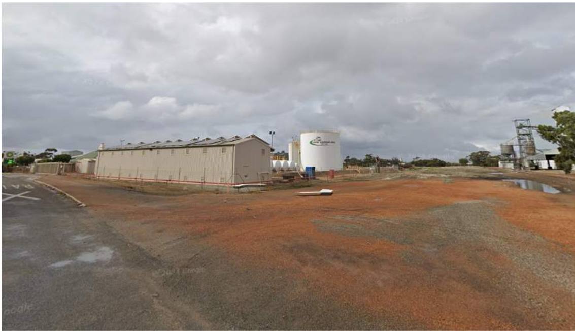
Figure 3 Looking east towards the subject site from Drove Street
