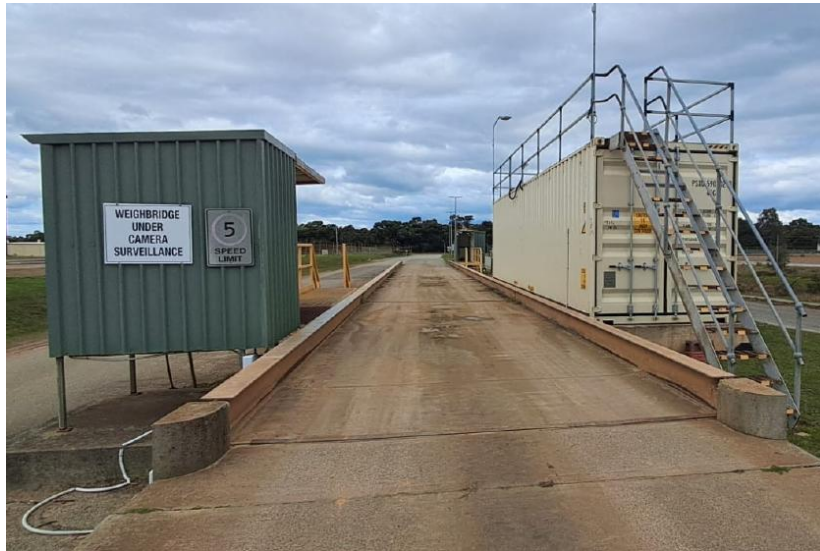
Figure example of weighbridge and sampling hut
