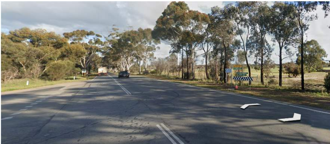
Figure 9 Henry Street T intersection with Gt Southern Highway
