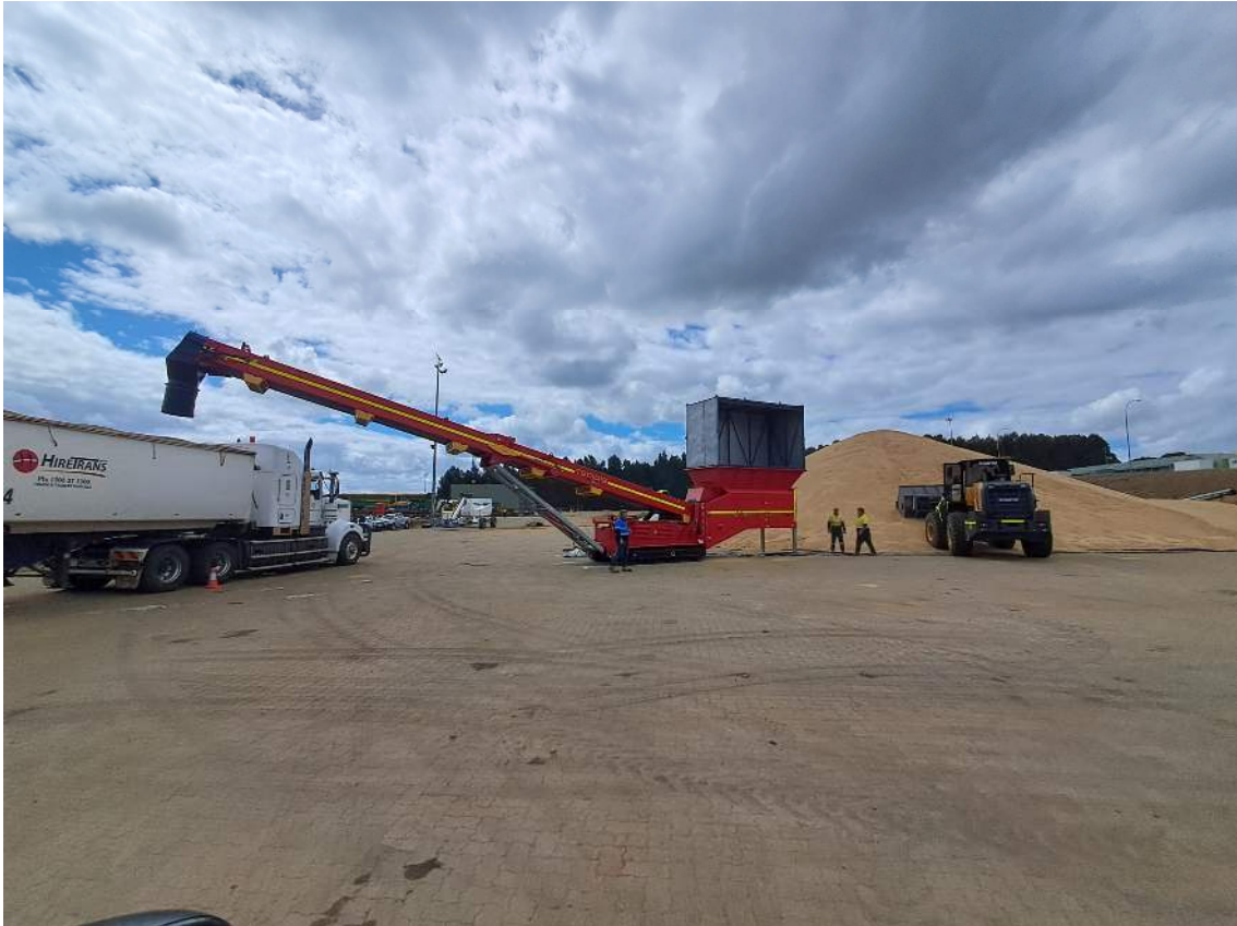
Figure 6 Mobile Conveyor in Operation Offloading Grain from a Stockpile
