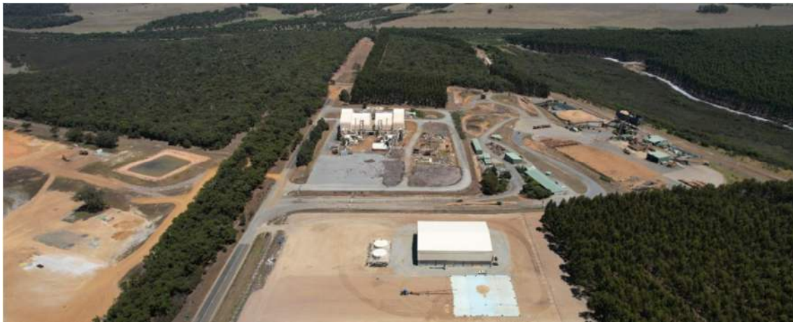
Figure 7 Commodity Ag's Downs Road Grain Handling Facility near Albany
